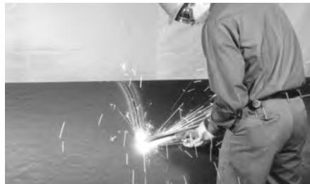
Cutting ductile iron pipe with torch.
