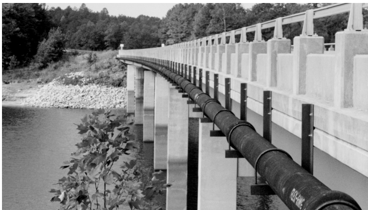
This bridge crossing illustrates design/construction advantages, including the deflection capabilities of AMERICAN Flex-Ring Joint Pipe.
