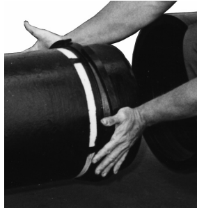
FIELD ASSEMBLY OF FLEX-RING
