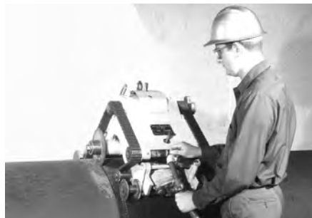
Cutting ductile iron pipe with milling cutter.
