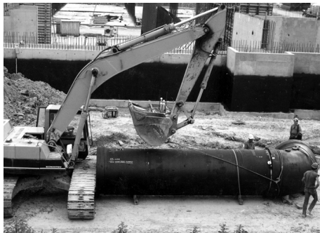
Assembly of a larger push-on joint fitting.
