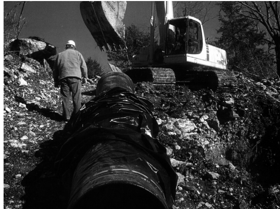
The versatile performance capabilities of AMERICAN Flex-Ring Joint Pipe are perfectly suited for projects containing a variety of conditions such as the hilly, rocky terrain shown in this photo.
