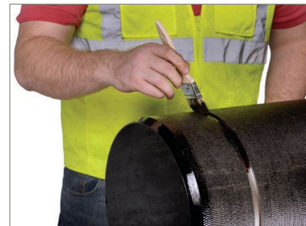
Preparing the pipe for installation of small diameter Field Flex Ring.
