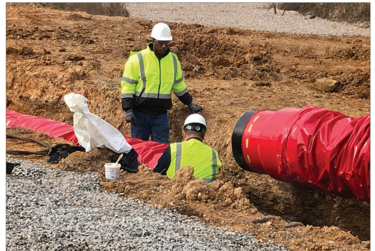
Joint assembly can be readily performed by two workers in a trench and one worker on the backhoe.
