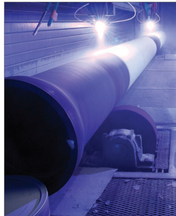
Metallized arc-spray application of zinc coating.
