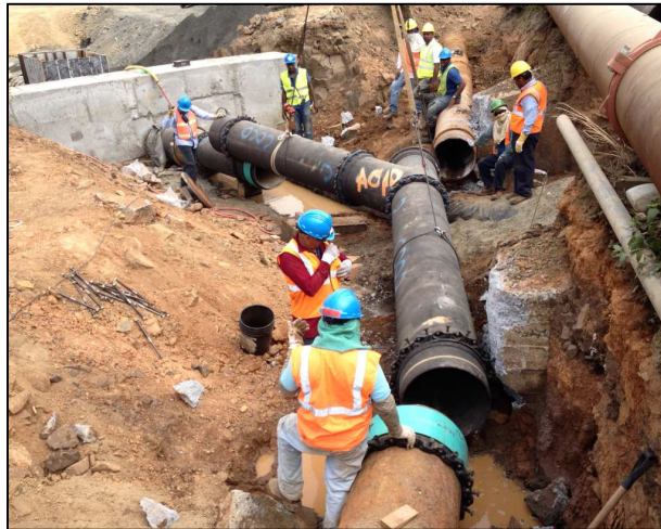
Figure 3: Thrust Block and Dielectric Coupling
