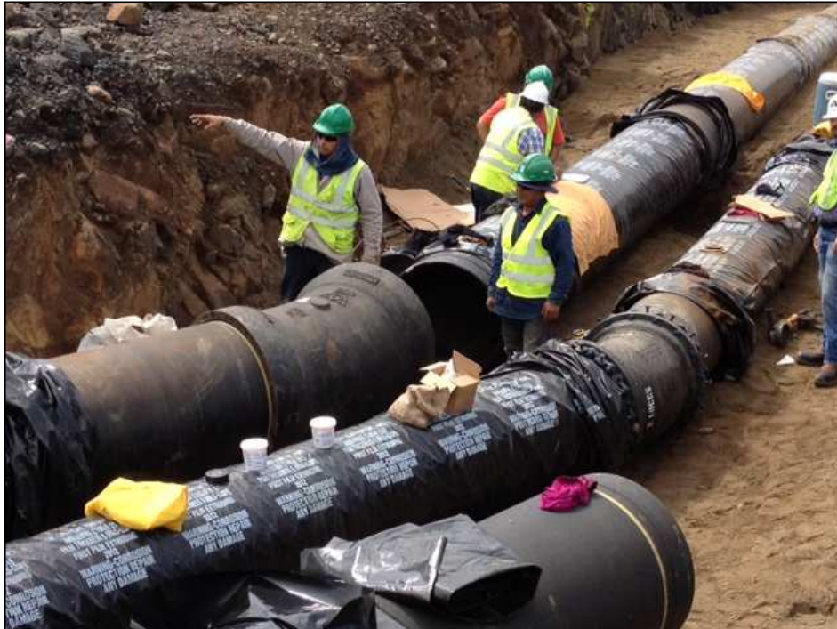
Figure 13: Installation of 30-inch and 24-inch Pipe at the Pacific Site
