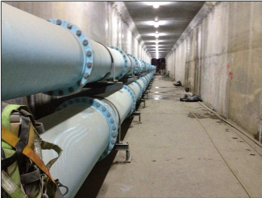
Figure 9: 24-inch and 30-inch Flanged Ductile Iron Pipe in Pacific Site Crossunder
