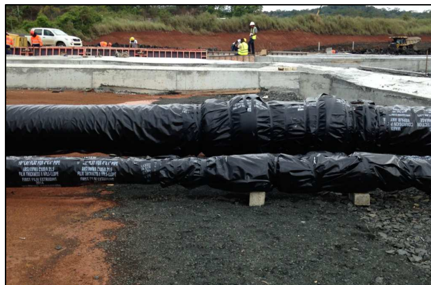
Figure 4: Flex-Tend Expansion Joints Encased in Polyethylene
