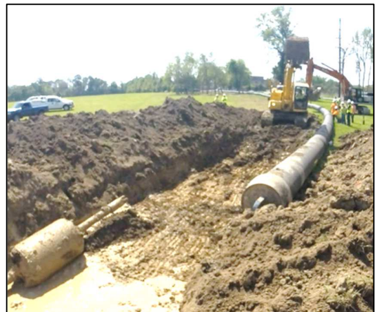
Figure 2 – Start of 740-Foot Pull
