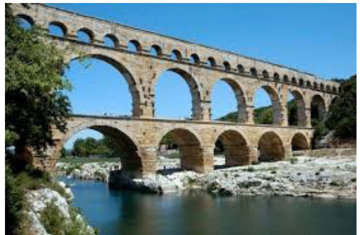
Figure 3. Roman aqueducts were necessary for the growth and security of the Empire.
