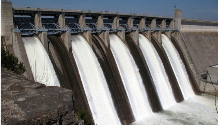
A hydroelectric dam producing power from river flows.
