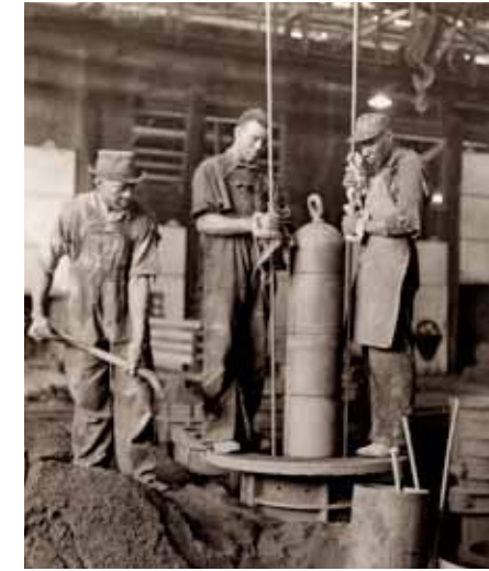
Workers ram pipe flasks by hand at the original ACIPCO foundry early in the 20th century. Part of the laborious pit casting system used before mechanized casting was introduced in the late-1920s, molding sand had to be shoveled into the flask and tamped with log rods a bit at a time to fill the space between the flask and the metal.
