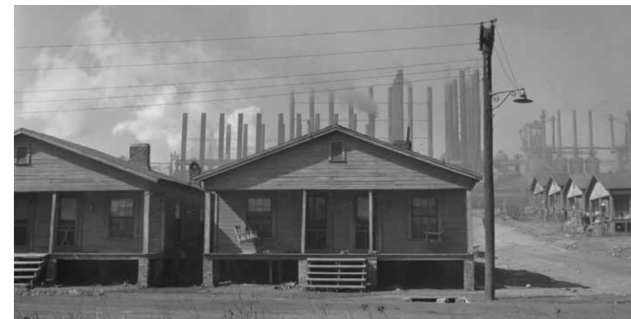
Steel and iron workers homes in the 1930s. Primarily constructed for black employees, industrial plants built housing near the grounds, cutting down on the challenges of accessing the plant, which many poorer workers had to do by foot.
