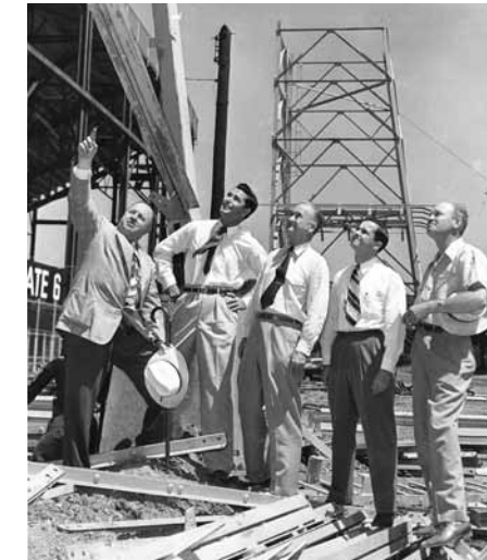
O'Neal Steel executives, including Kirkman O'Neal (third from left) and his son Emmet O'Neal (fourth from left), during the construction of the upper deck of Legion Field in 1961.
