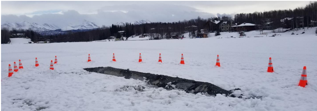
Figure 3. The highest-elevated joints rising through the ice on March 14, 2019, 104 days after the event.
