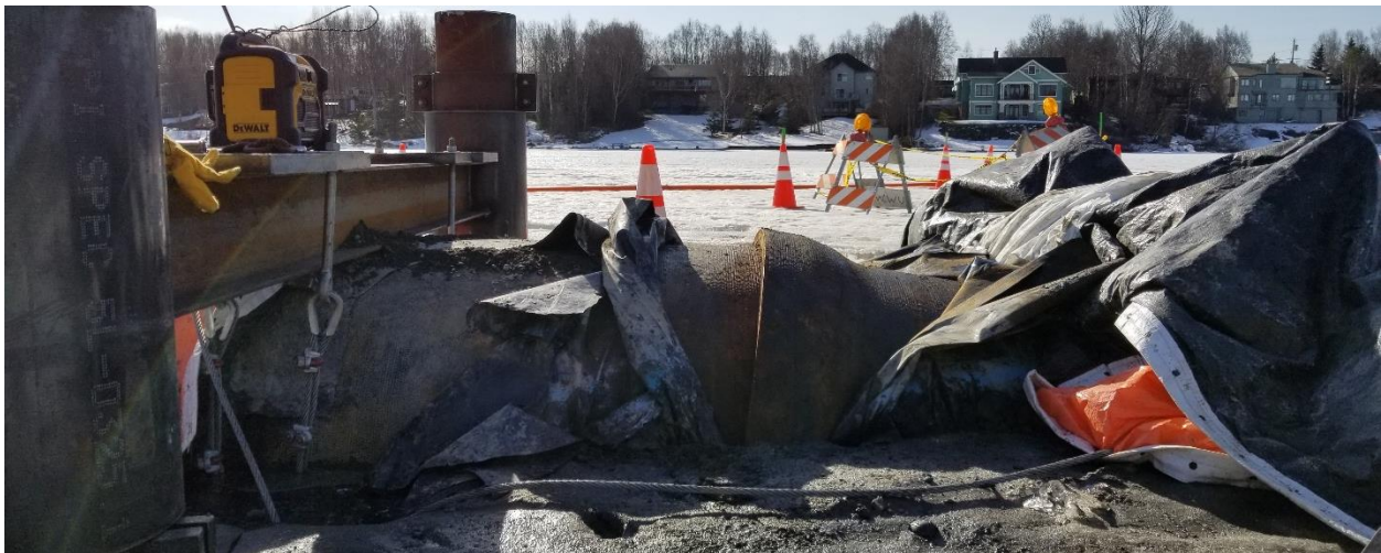
Figure 5. A Fastite push-on joint ductile iron pipe deflected at a calculated angle of 14-degrees and maintaining joint performance.
